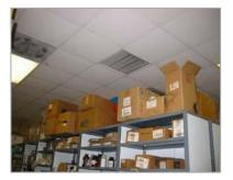
These items are stored too close to the ceiling. In an area without a sprinkler system, the fire code states that there must be a 24-inch clearance between the ceiling and stored items.
