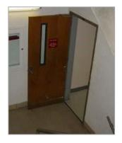
In a fire, stairwells with fire doors propped open to act as chimneys allowing fresh air to reach the fire. An open door allows the smoke and fire to spread to other floors quickly.
